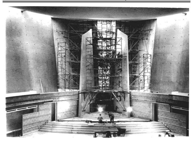
Temple Beth Zion – Building Construction; workman finishing bimah and Decalogue pylons (November 4, 1966)
